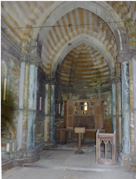
Figure 6: Interior walls and vault lined with contrasting marble.
